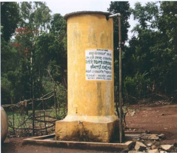
Figure 3: Water tank with 10,000 liter capacity
