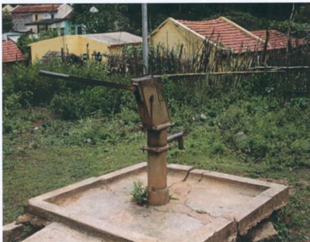
Figure 4: Closed bore well with hand pump
