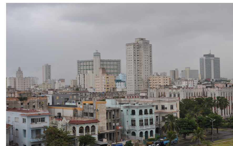
Figure 2: Vedado, showing the earlier Republican period buildings in the foreground and the suburb's modern development in the background. Wikipedia Commons, 22 April 2017.
