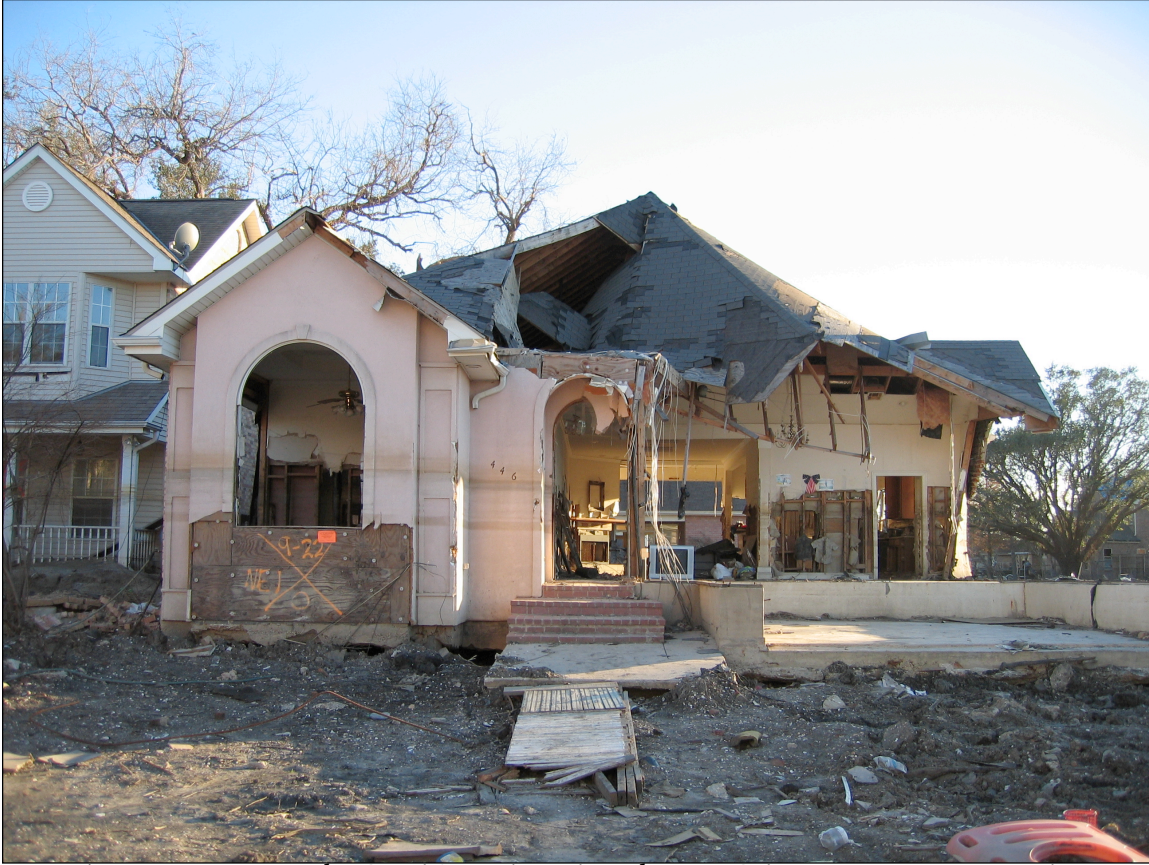
Figure 8. House near the Canal Street levee breach, New Orleans, Louisiana, December 2005. Photo by the author.
