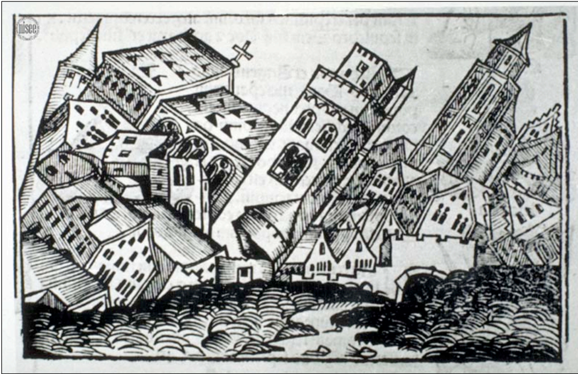
Figure 2. Medieval illustration of biblical earthquake (1493). Courtesy of the National Information Service for Earthquake Engineering, EERC, University of California, Berkeley
